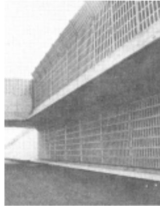
Fig.6 Example of top-bent barrier.
